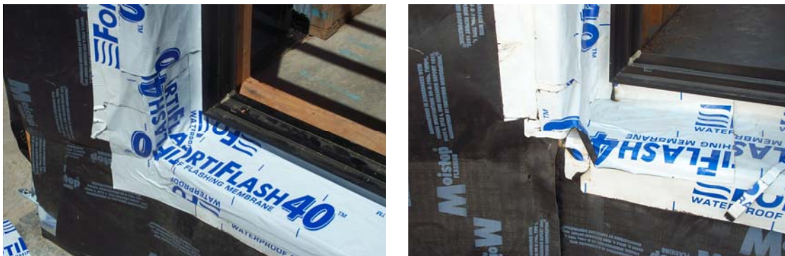
Figure 7 Exterior sill flashing of a recessed window using self-adhered flexible flashing. Multiple layers are required to fashion corners, resulting in wrinkles and fishmouths. Voids behind inside corners are vulnerable to puncture
