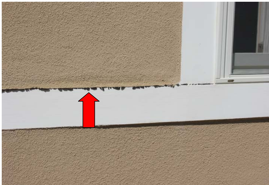
Figure 12 Adhesive polymer from a self-adhering flexible flashing flowing out of a joint between wood trim and stucco
