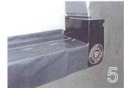
5 With both CAPs in place, install SAM to cover the sill completely, as shown. Form the back dam of the sill pan by wrapping over the back leg of each CAP. If desired, remove the unused vertical portion of the CAP (flush with the jamb stud) to ease installation.
