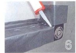
6 After creating the pan, install additional SAM flashing over the CAP at the jamb, as shown. Finally, add sealant to the inside corners where the two flashing pieces meet, to provide additional protection. Repeat these two steps at the opposite side's CAP. Install the window unit.
