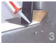
3 For extra protection, sealant may be applied to the edges of the WillFlash® CAPs just before installing.
