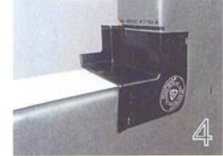
4 Position the CAP at the sill-jamb condition. If sealant is used, press down gently to ensure contact with substrate materials. Secure the CAP with fasteners. Repeat all of these previous steps to install a CAP at the opposite sill-jamb condition. Clean surface of CAPs to receive self-adhering membrane (SAM).
