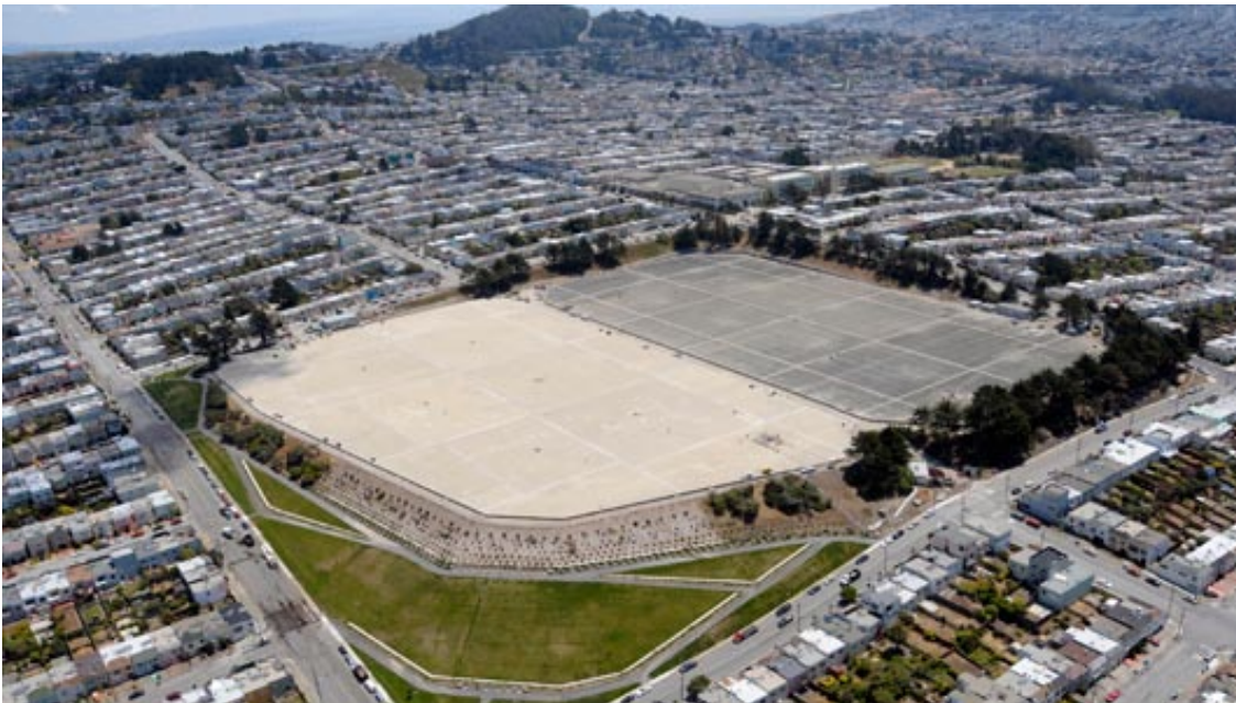
Current aerial view of the eight-block reservoir in San Francisco's Sunset District where 25,000 solar panels will soon be installed.
