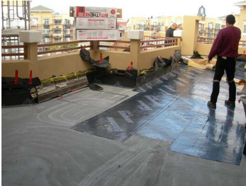
Figure 12 Sloping mortar substrate over wood deck sheathing
