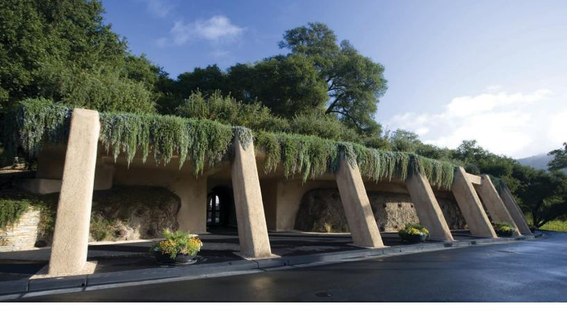
steel rock anchors, driven fifteen to twenty-five feet into the bedrock. The finish of the structure is a spray-applied mixture of cement and earth called PISE (Pneumatically Impacted Stabilized Earth). The structure was designed to integrate into the hillside to minimize erosion and provide stability. The cave roof also doubles as a planting bed for native grasses and other drought-tolerant plantings.
